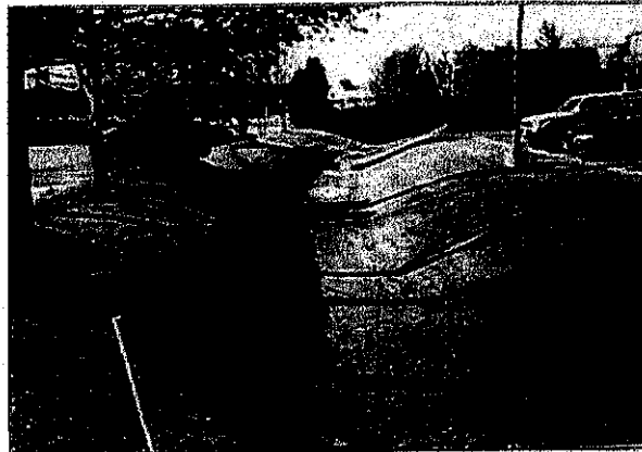
This dry swale is located in New Hampshire. It blends well with the landscaping and is low maintenance yet effective. It does have an overflow to the storm drain system that can be accessed once the water reaches more than halfway up the side slopes.
